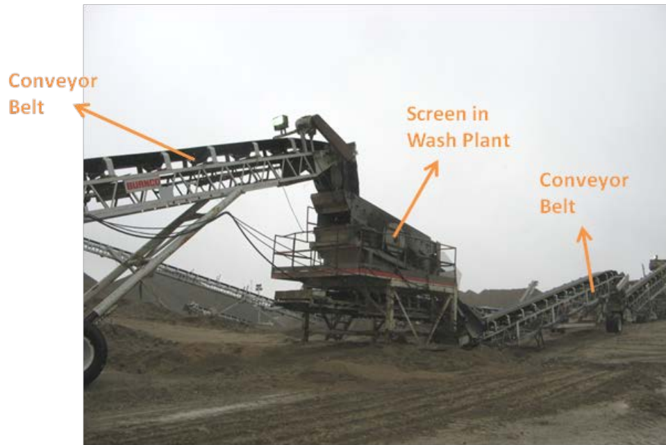
Photo 5: Screen 3 in the Wash Plant
